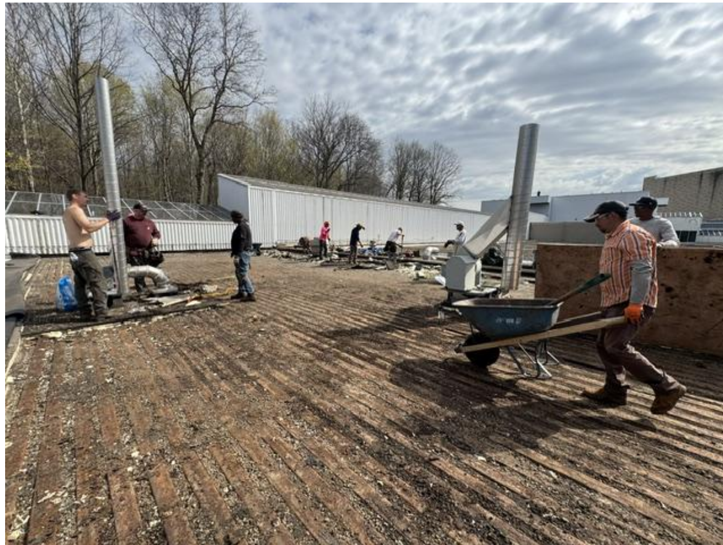
► Roof Replacement Project
