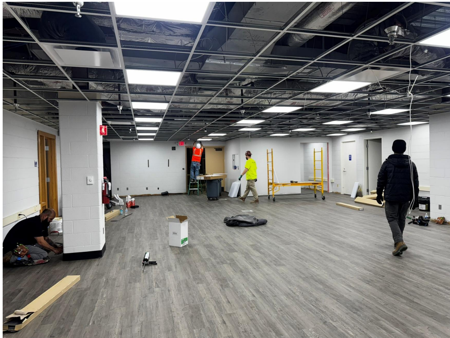
► Early Middle College Renovation Project
