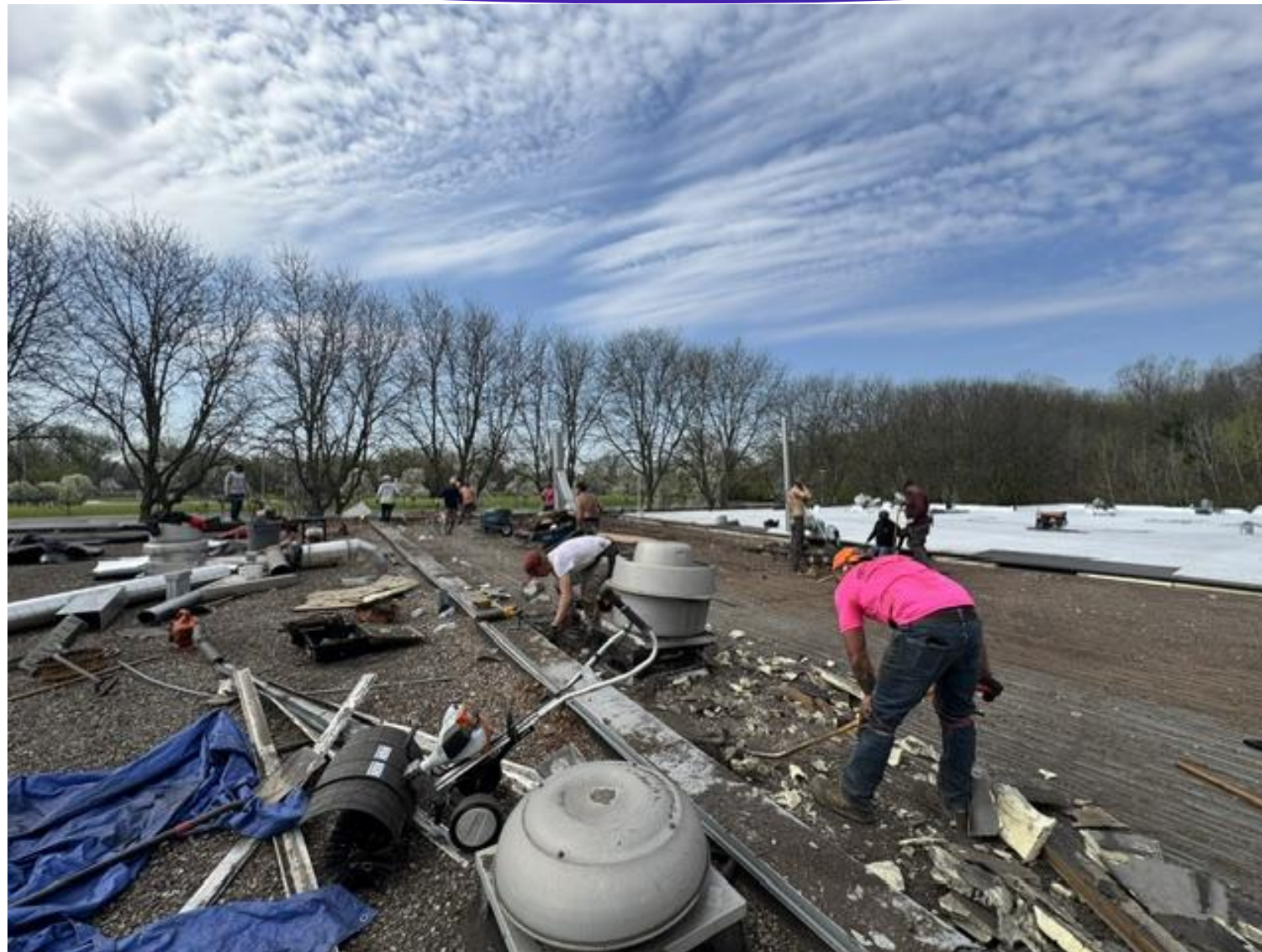
► Roof Replacement Project
