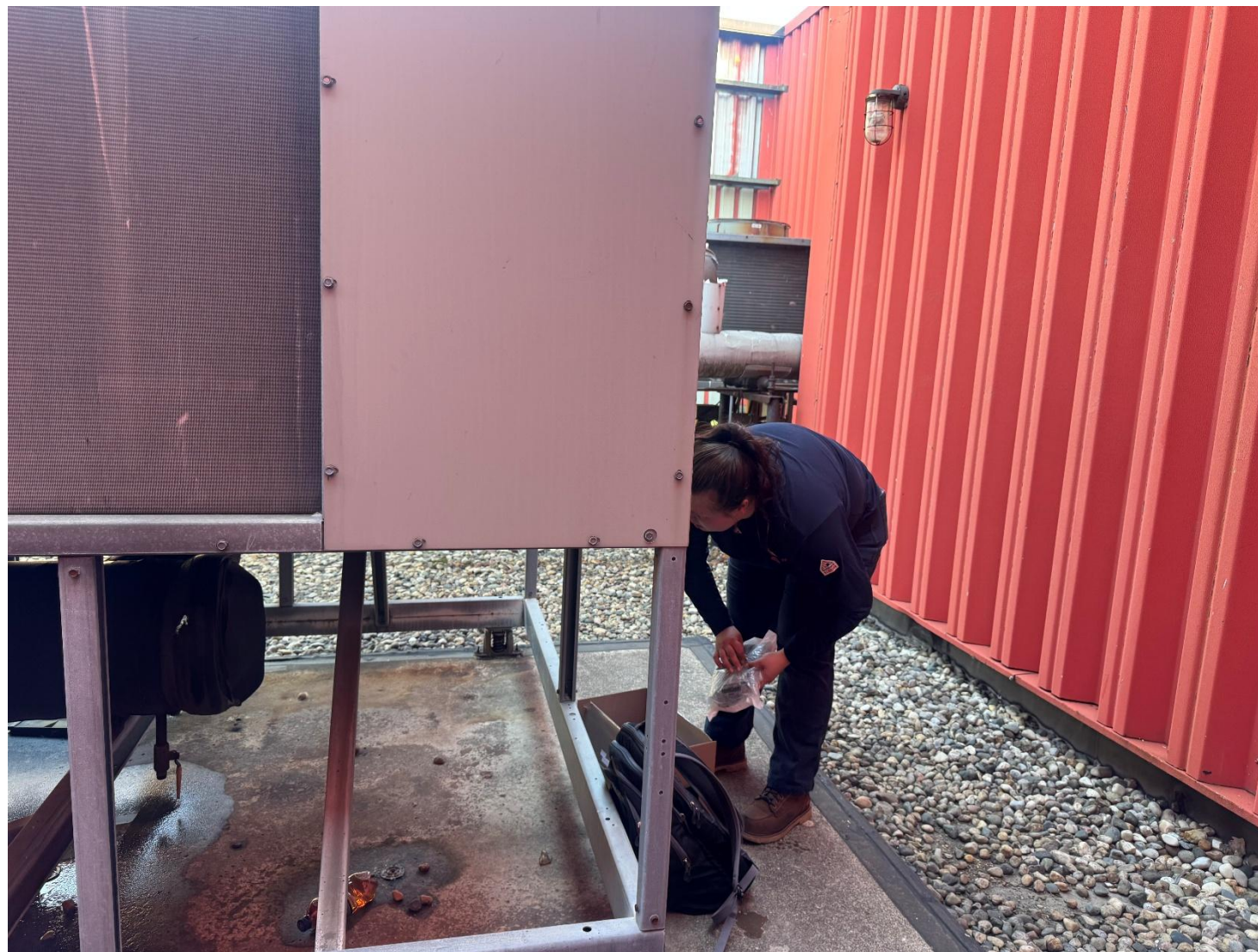
► HVAC Repair Project
