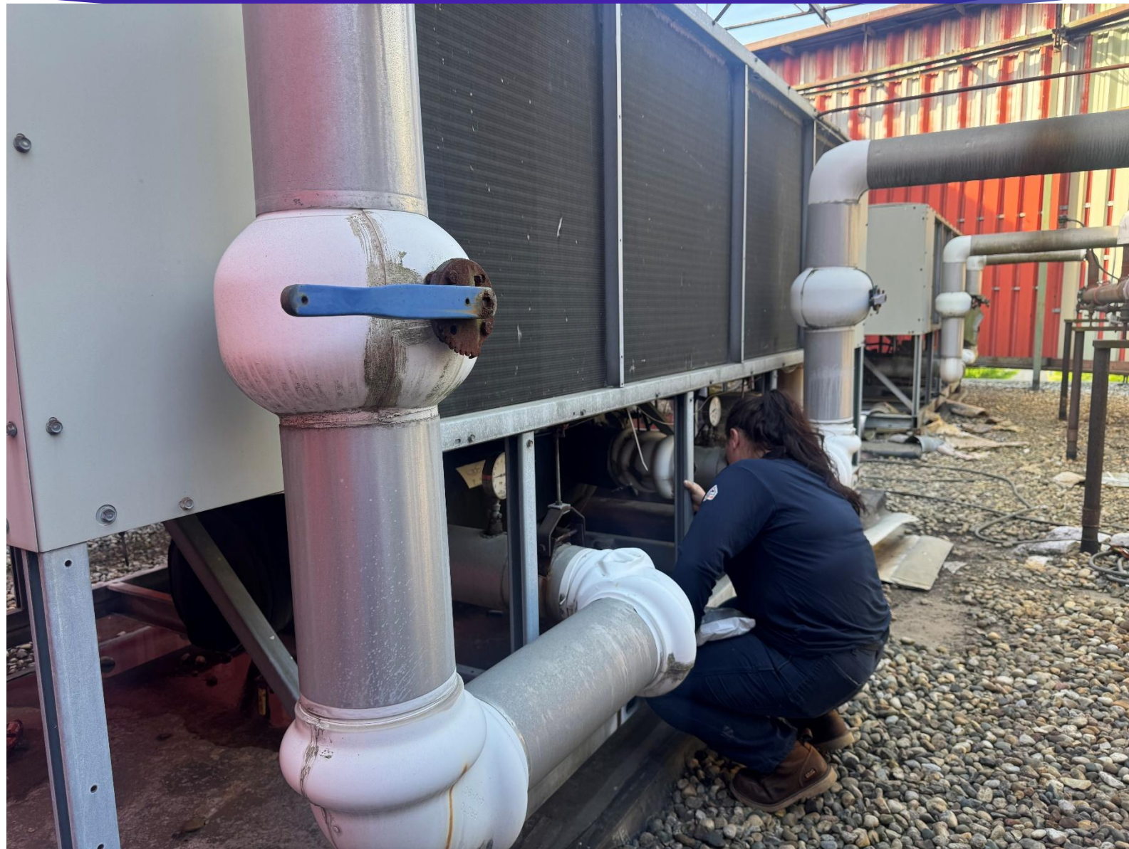
► HVAC Repair Project
