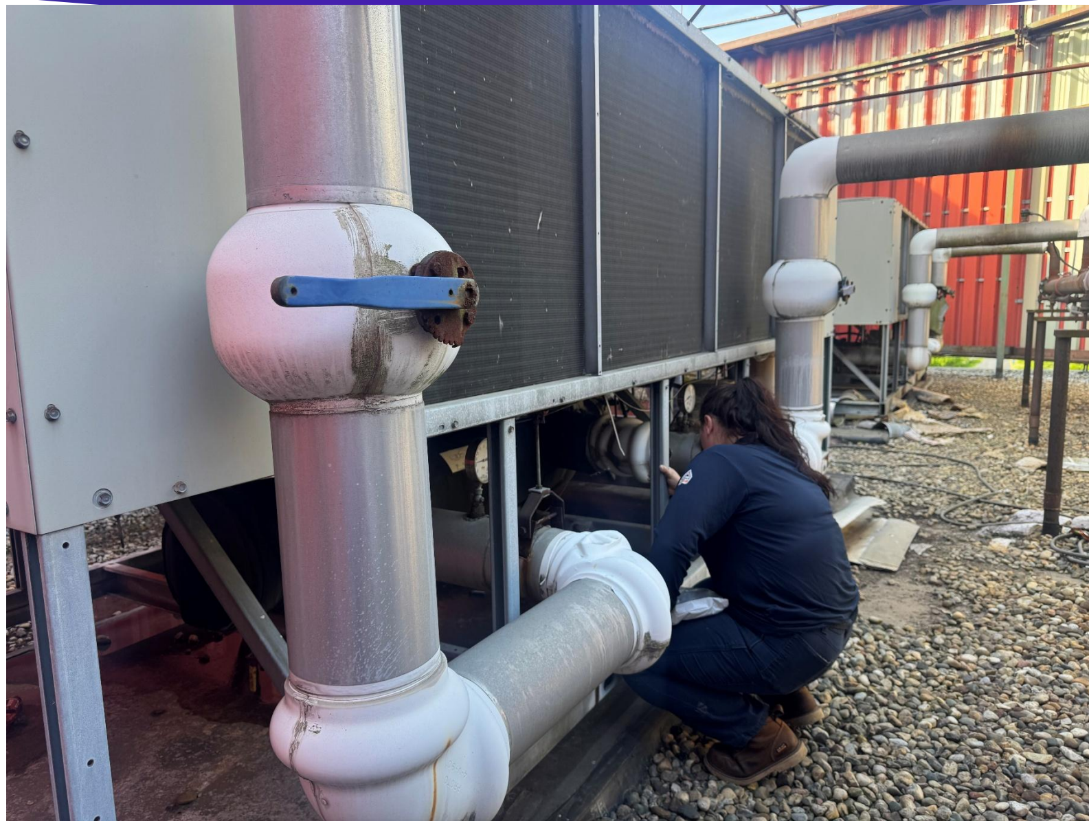
► HVAC Repair Project
