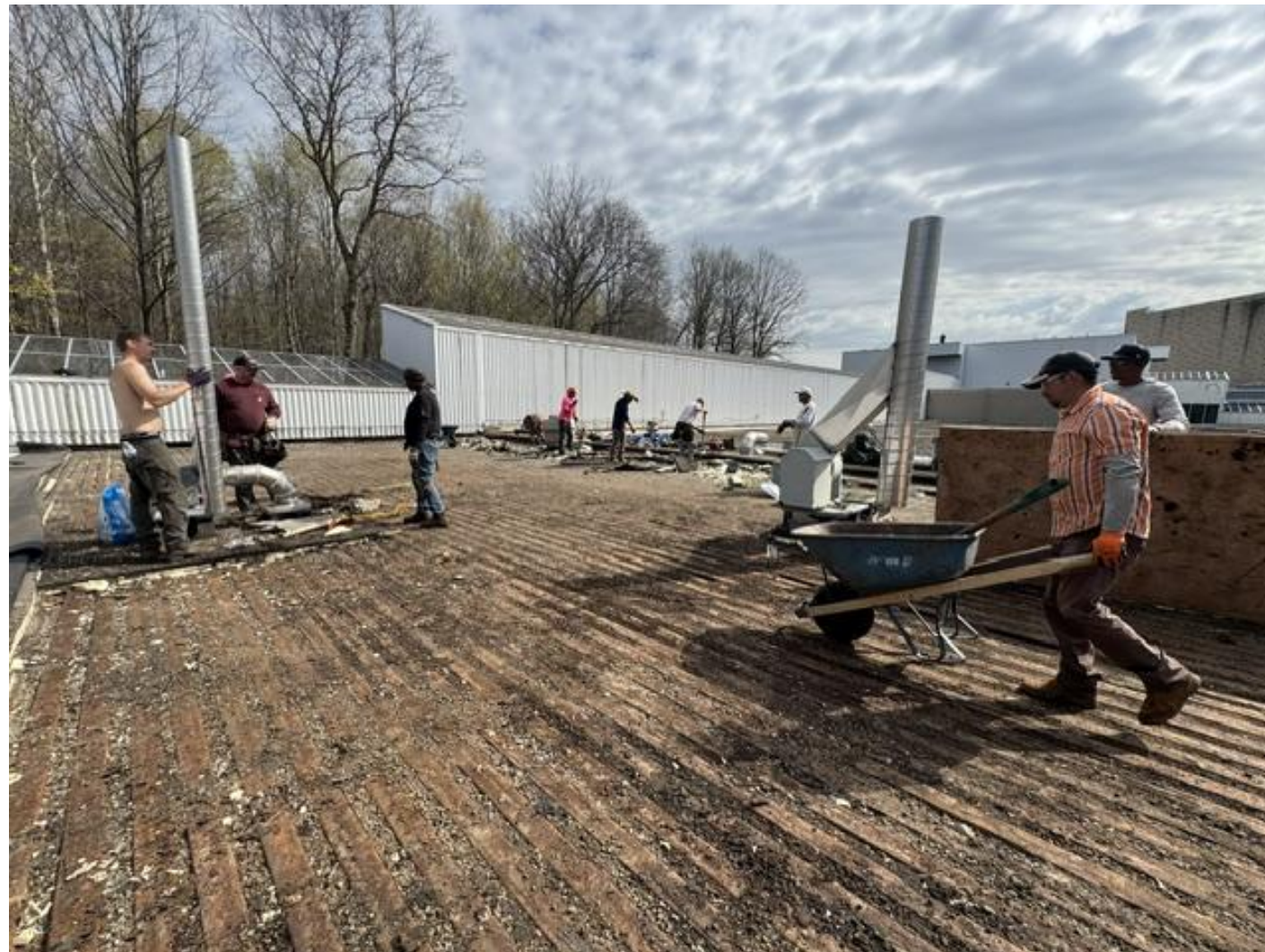
► Roof Replacement Project
