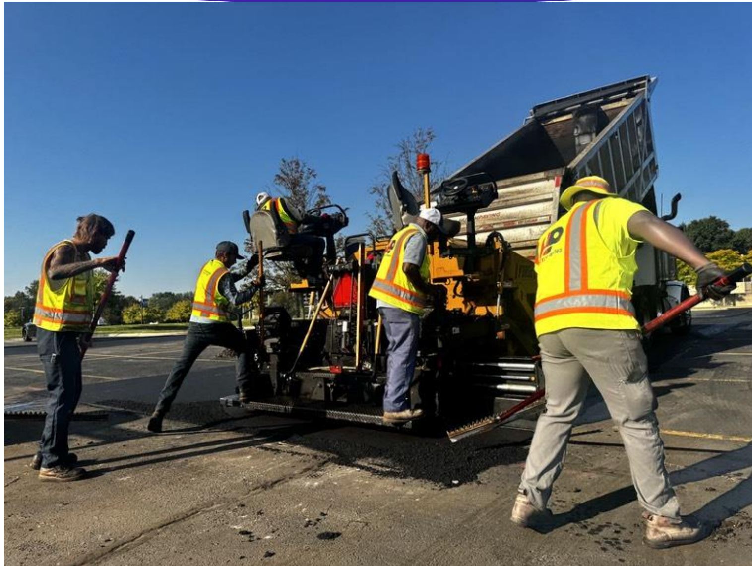
► Pavement Maintenance Program Project
