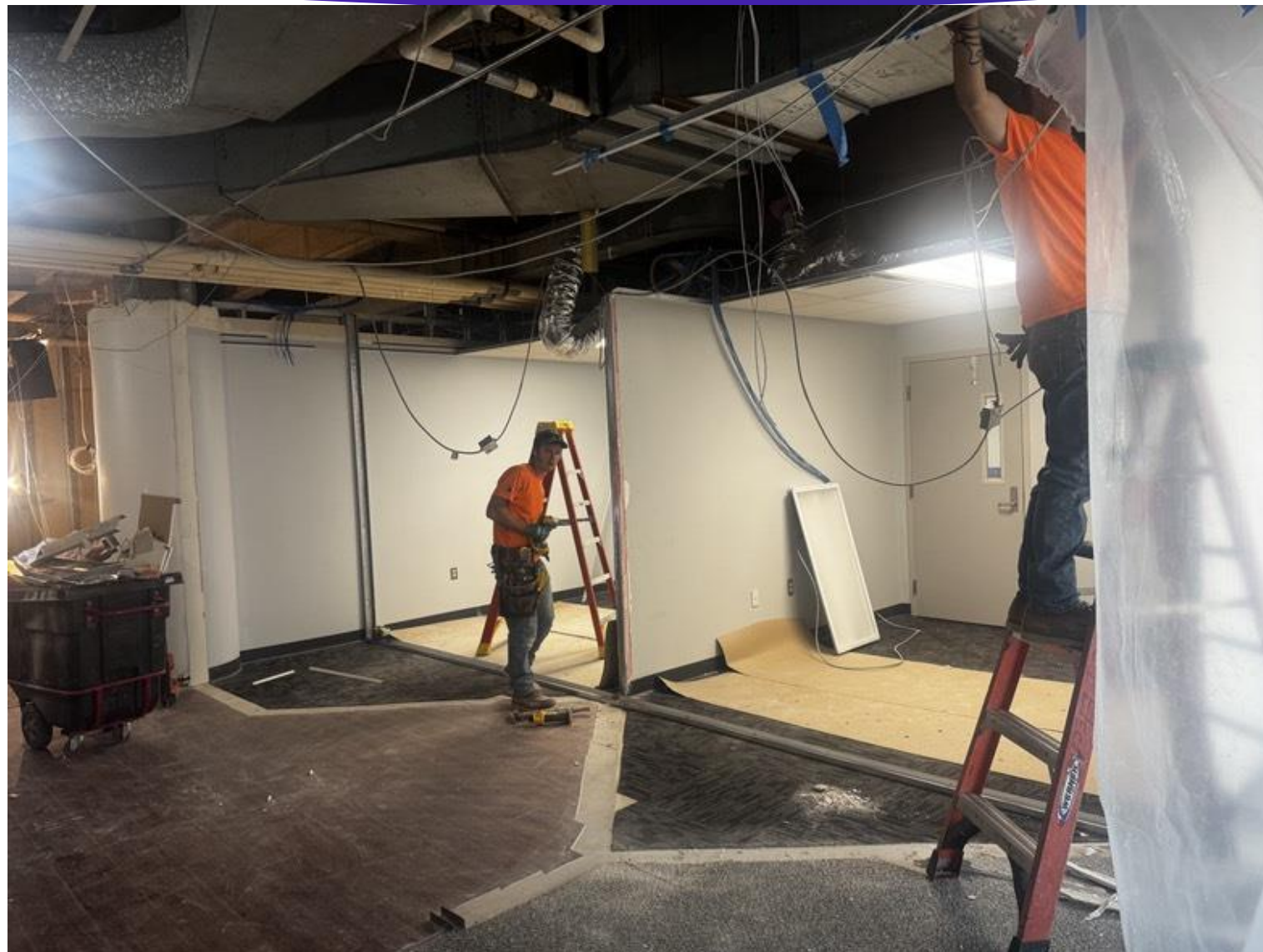
► 5 th Floor Improvements Project
