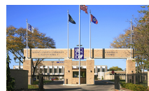
NORTHWEST CAMPUS 8200 W. Outer Drive Detroit, MI 48219 313-943-4000
