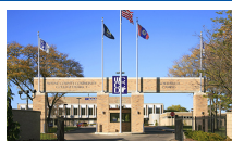
NORTHWEST CAMPUS 8200 W. Outer Drive Detroit, MI 48219 313-943-4000
