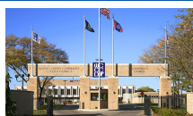
NORTHWEST CAMPUS 8200 W. Outer Drive Detroit, MI 48219 313-943-4000
