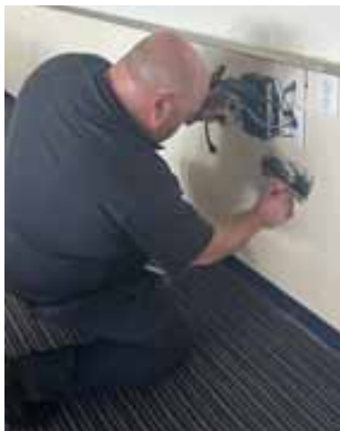
Repairing and reinforcing interior walls.
