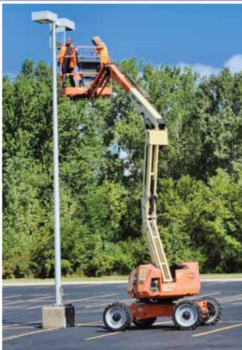
Replacing parking lot lights
