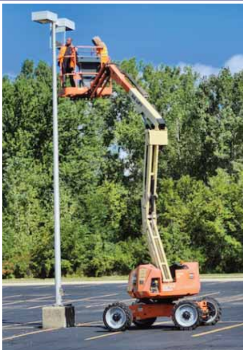
Replacing parking lot lights
