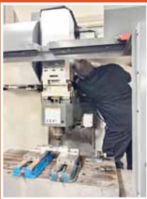
Computer Numerical Control (CNC) Machine Installation
