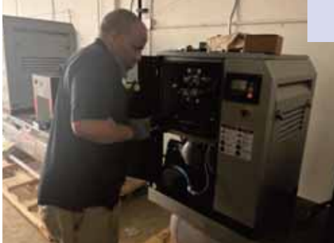
Air Compressor Power installation
