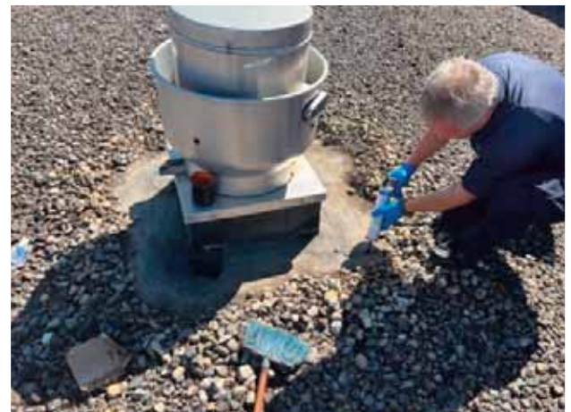
Roof Leak Repair
