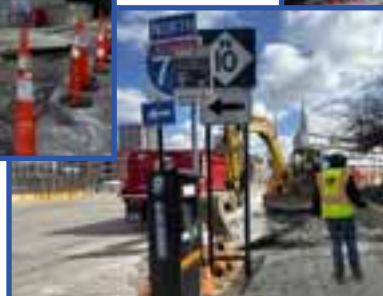
Executive parking lot and sidewalk repairs continue.
